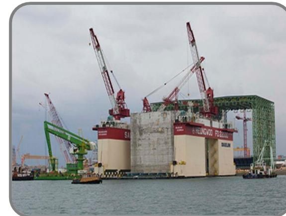
Reduced construction time using floating docks
