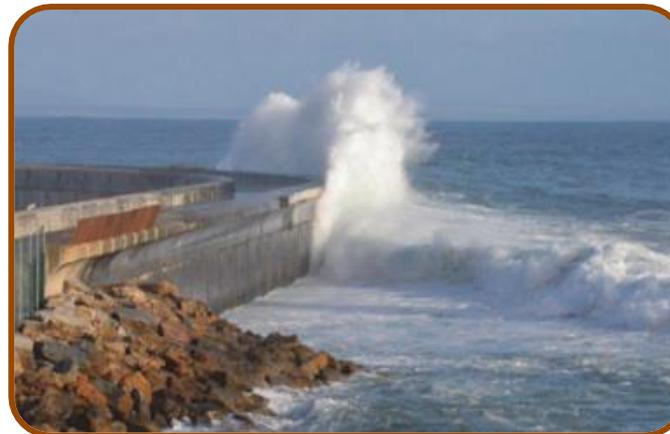
Provide sufficient weight to withstand wave forces
