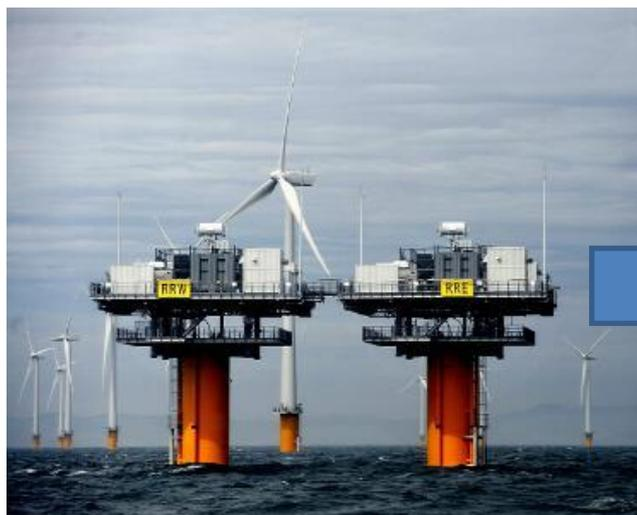
Currently, the most common solution is similar to the WTG foundations with substations over monopiles/jackets
